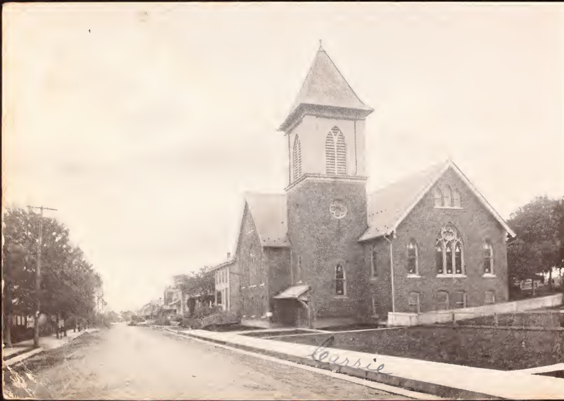
THIRD STREET, LOOKING SOUTH FROM LUTHERAN CHURCH,
